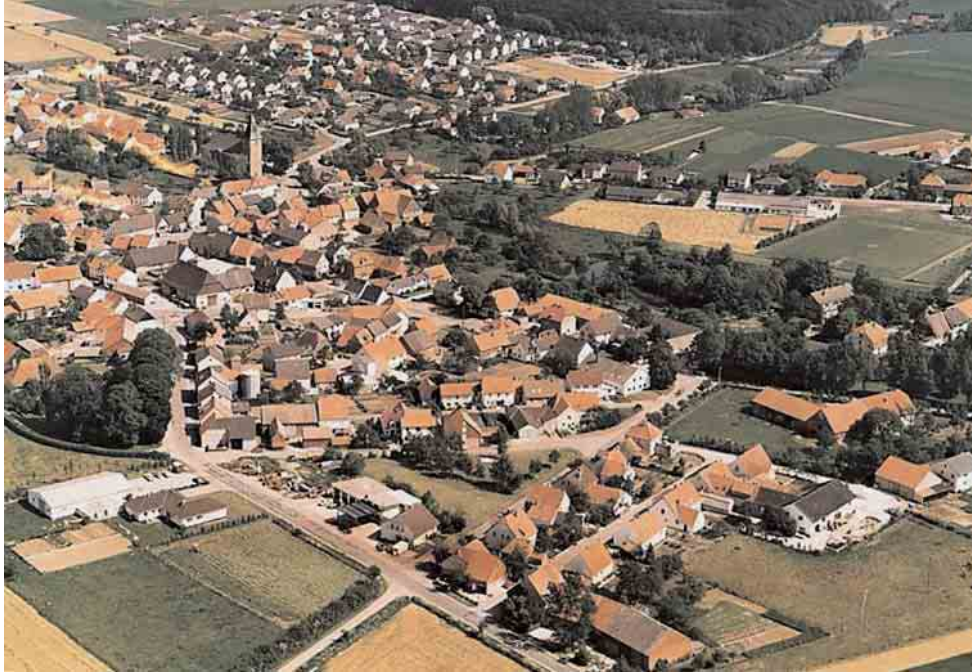
The George Lenz farmhouse was located on the outskirts of Bühne. The road leading off the bottom center of the above photograph is the one on which the farmhouse was located. A new house has replaced the old one, which was destroyed by the bombs of WW II. Farming fields can still be seen in this 1981 photo of Bühne.
